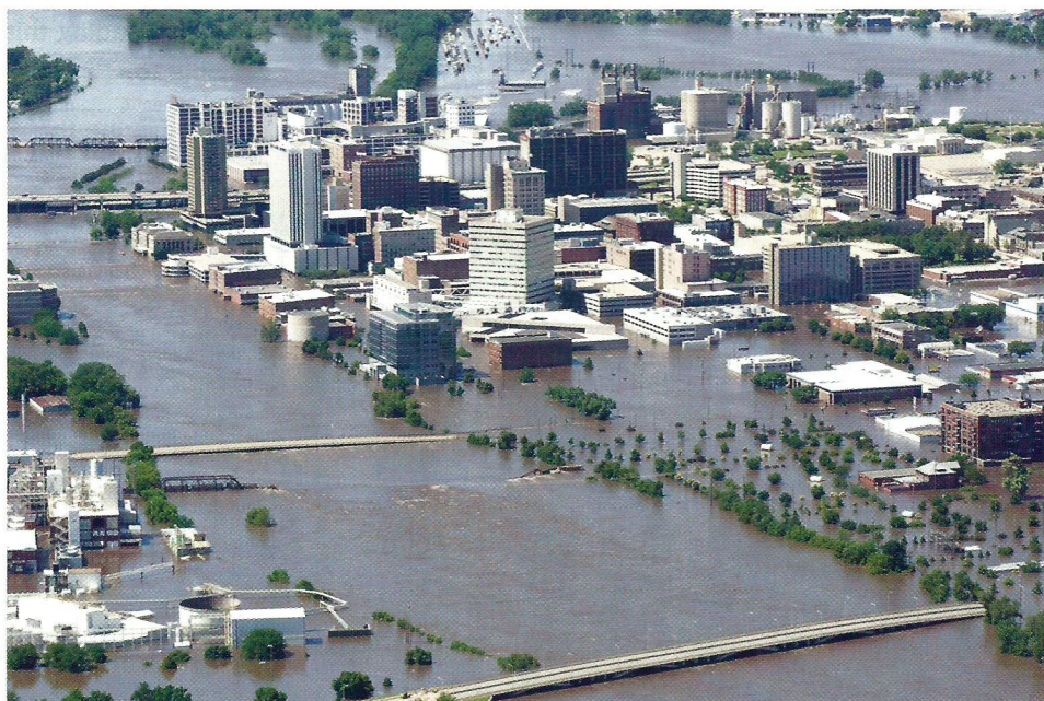
▲ FIGURE 7-2 Flood damage at Cedar Rapids, Iowa, June 2008.
