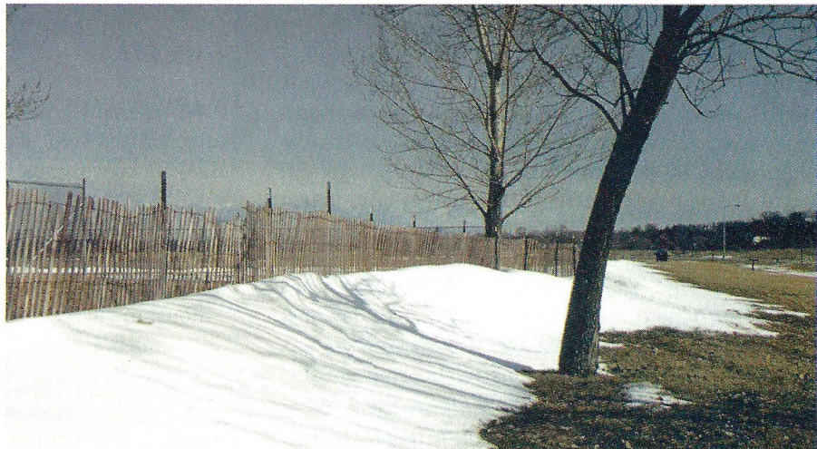
FIGURE 9.9 A snow fence slows the wind, thereby decreasing the wind's ability to transport snow. Hence, snow accumulates to the lee of the snow fence. [Photograph by J. M. Moran]
