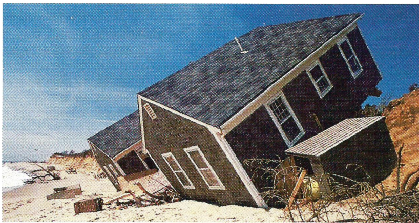
A house tilts as sand is eroded from the beach and cliffs ( left background ) by storm waves. Nantucket, Massachusetts. (Steve Rose/Rainbow.)
