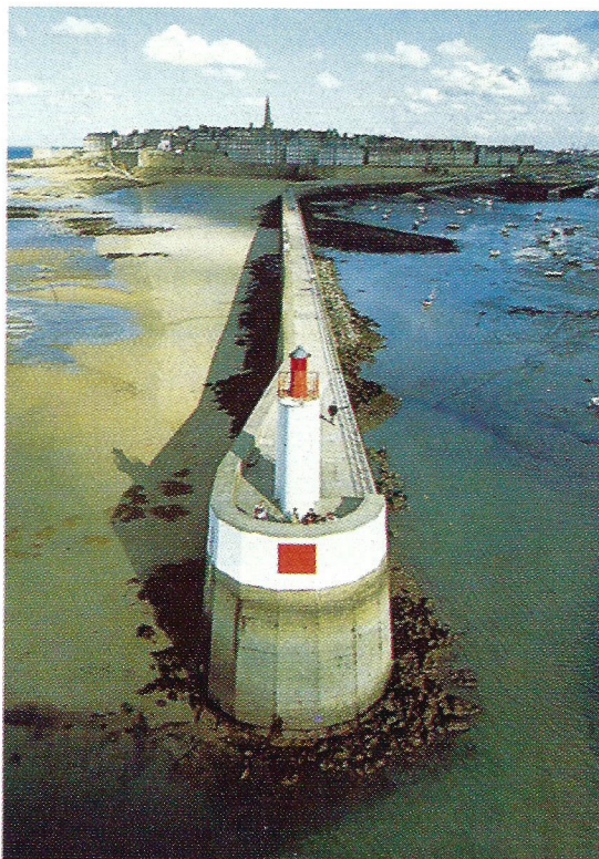
Construction of groins along a shore to control erosion of a beach may produce erosion downcurrent of the groin and loss of parts of the beach ( right of groin ) while sand piles up on the other side ( left of groin ). Longshore current flows from left to right. (Philip Plisson/Explorer.)
